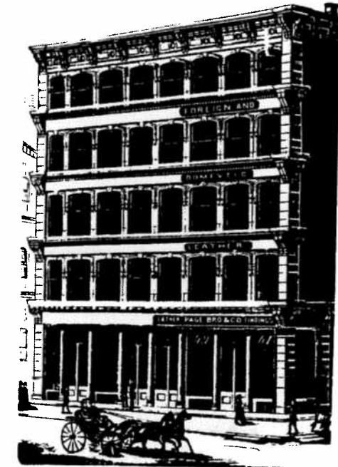
Two of the few surviving examples of post-Fire commercial buildings in the Loop: the Page Brothers Building (above) and the Delaware Building. Both are designated Chicago Landmarks.
